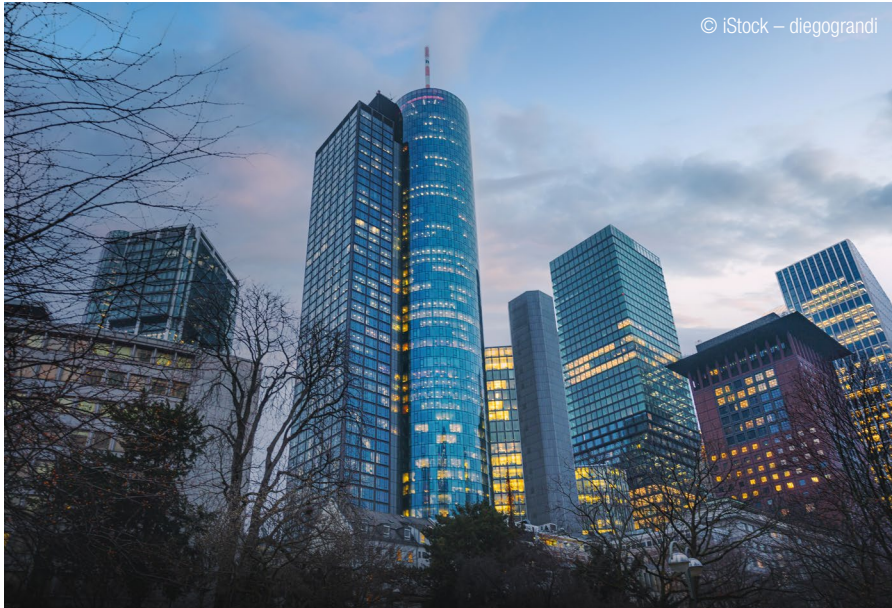
The MAIN TOWER is part of the Frankfurt am Main skyline. In 2022, a comprehensive modernization of the building control system as well as the building and room automation was started.
